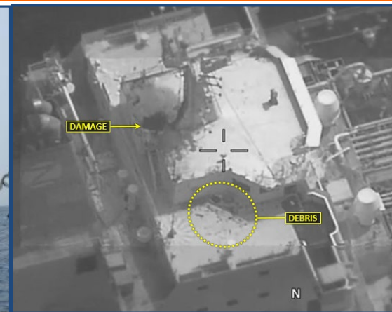
(U) Damage Caused by Iranian UAV Attack
